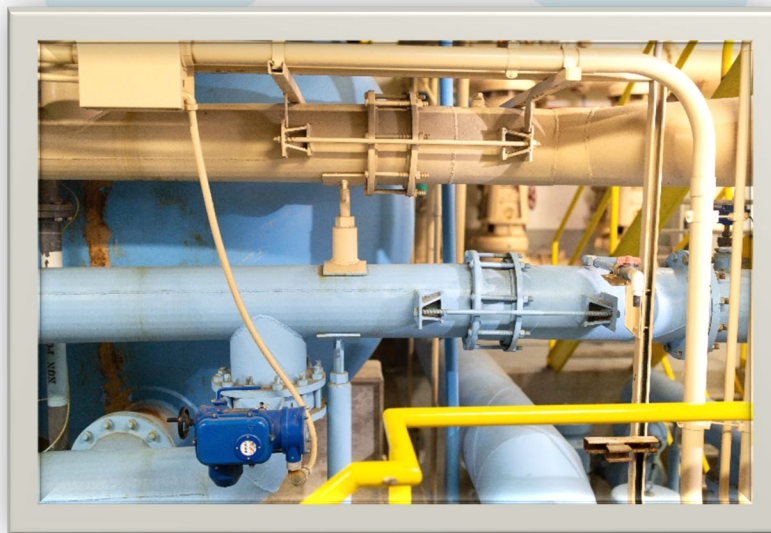
Wastewater treatment facility tri-media filter, pipes, fittings, and valves.
